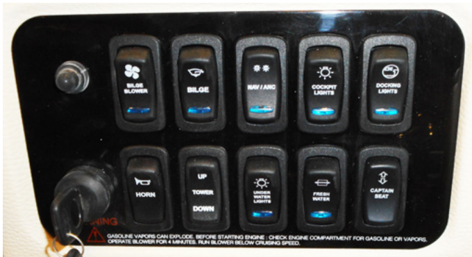
Typical Switch Panel Shown
