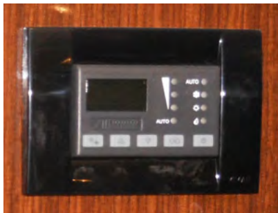
The Elite control panel (thermostat).
