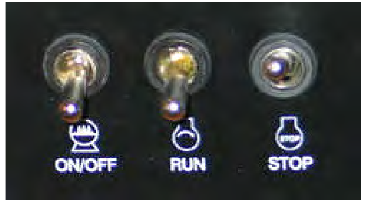
TYPICAL GEN-SET SWITCH CLUSTER- MAIN PANEL
