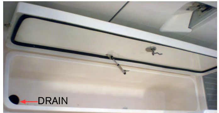
TYPICAL FLOOR STORAGE LOCKER
