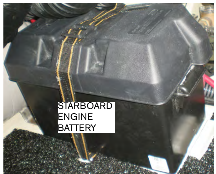
STBD AFT DECK
