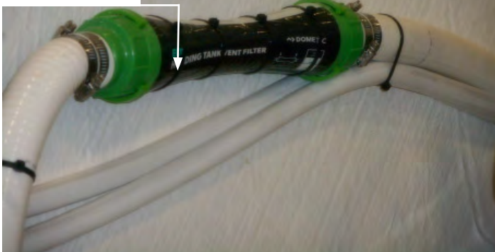
Typical Waste System In-Line Filter
