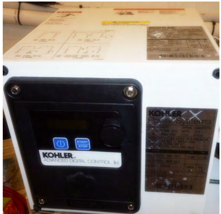
TYPICAL GEN-SET REMOTE ELECTRICAL PANEL
