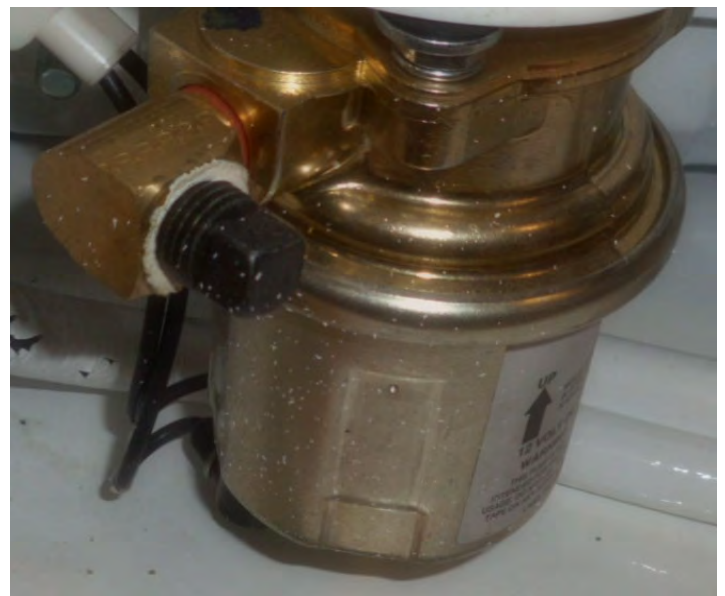
TYPICAL GENERATOR INTEGRATED FUEL FILTER
