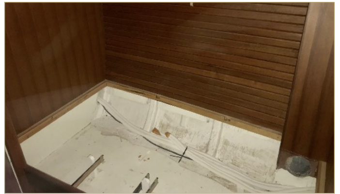
Port cabin under construction
