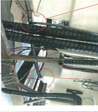
1 1/2" Scupper Drain 90° Elbow Hose Size: 1 1/2"
