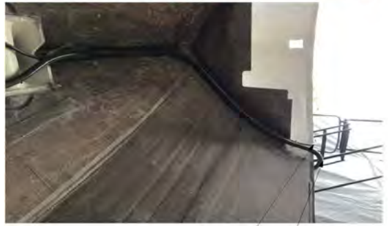
To Water Fill Cap (On Deck) To Water Tank Vent (On Deck)
